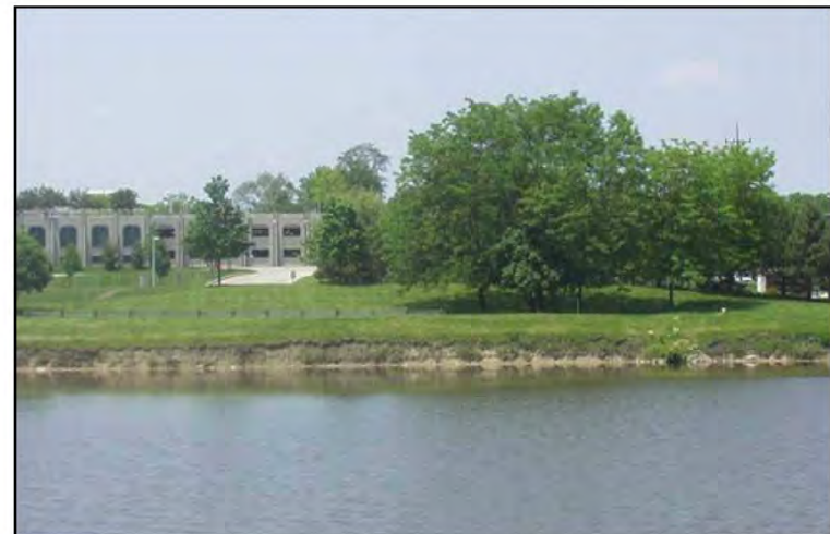
Photo 4 – View of stormwater pond lacking shoreline vegetation and showing erosion on the lower slope where turfgrass has failed.
