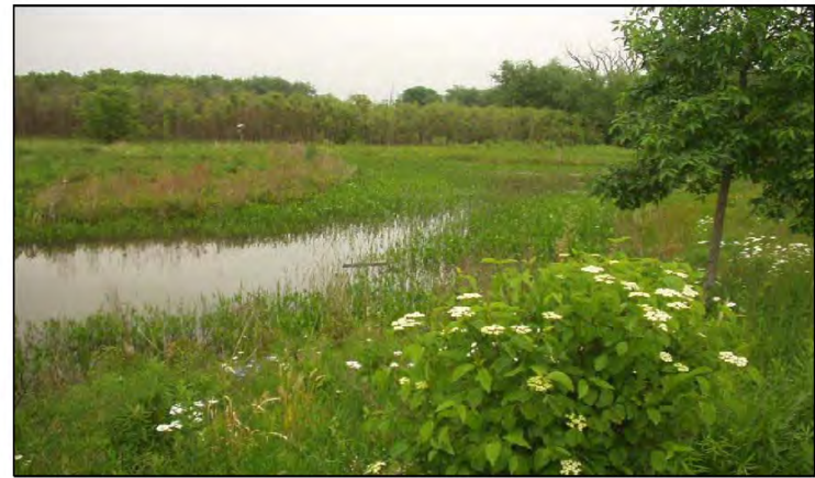
Photo 8 – Wetland bottom basin with broad emergent shelf and wet-mesic prairie slopes with clusters of woody vegetation. Note the irregular shape of the basin and the habitat nest box in the background (early summer).
