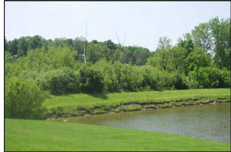
Photo 2 – View of stormwater wetland pond. Note the slumping associated with the basin margin due to shallow roots of the bluegrass turf.
