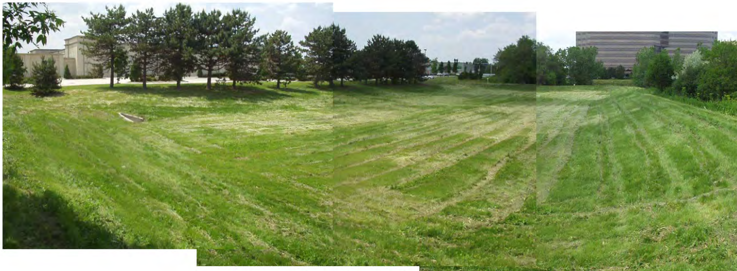
Photo 5 – View of dry bottom detention facility with mowed turfgrass. This type of basin does not offer the range of water quality and habitat benefits provided by a wetland bottom stormwater facility or a wetland pond. Turfgrass basins also have a high cost for maintenance over the life of the basin.
