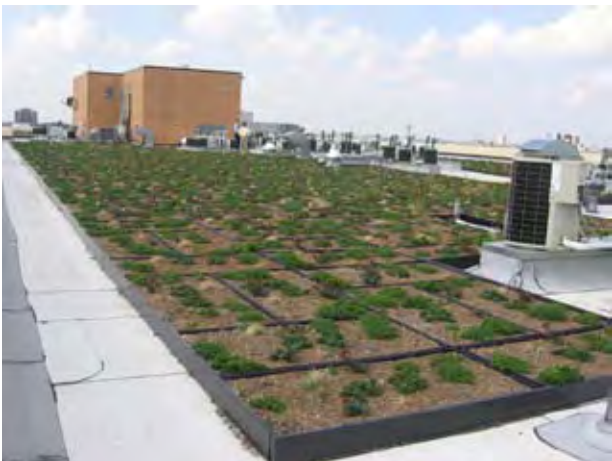
Green roof systems can reduce the ultimate heating and cooling costs of a building while providing a reduction in stormwater quantity at the source, the roof.
