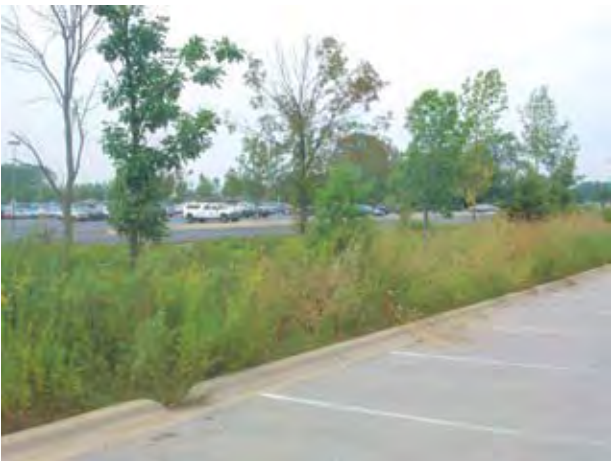
Using bioswales and level spreaders, in coordination with permeable paving, can result in a dramatic reduction in the amount of stormwater that eventually makes it to the storm system.
