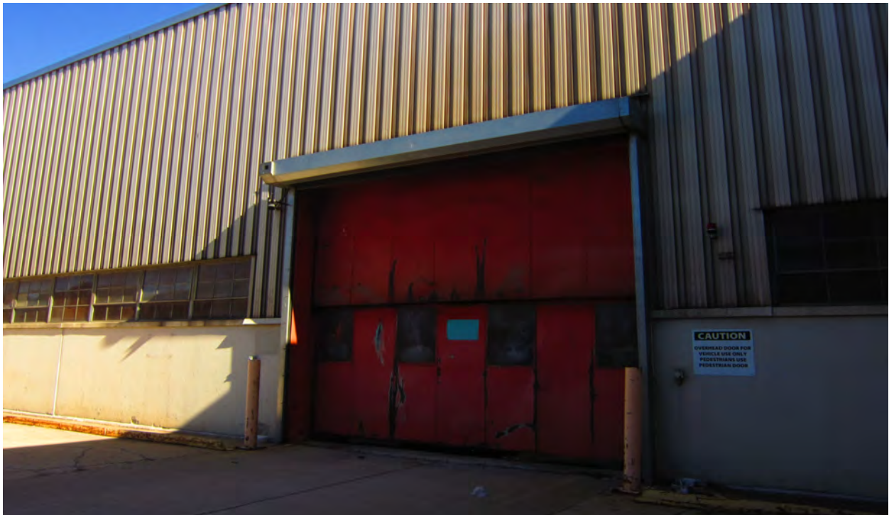
Example of damage to loading bay doors, and broken windows.
